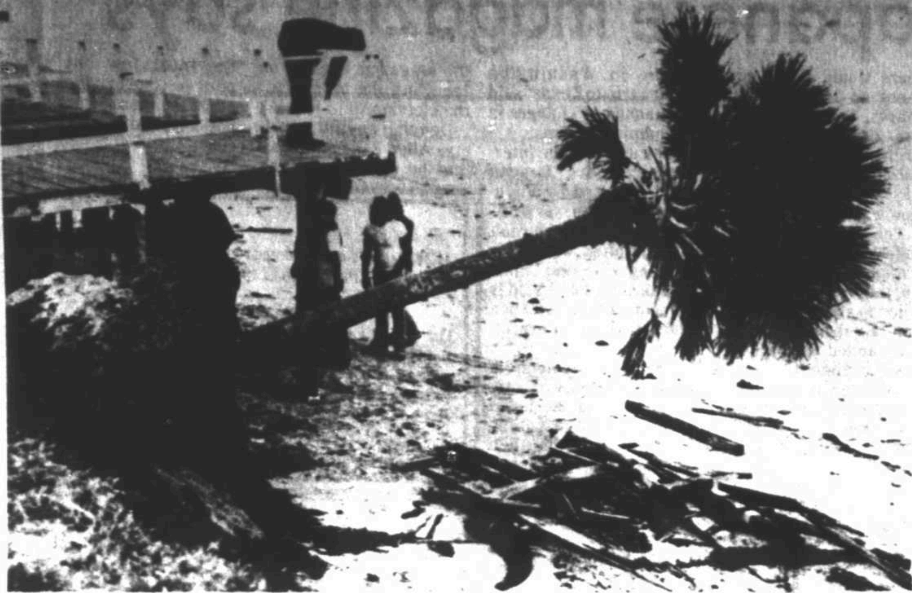
Two palm trees were toppled, a 100-foot sea wall crumbled and eight to 12 feet of ground disappeared into a hungry Atlantic Ocean Saturday at Ocean Star Motel and Apartments in Cocoa Beach, Fla. High
