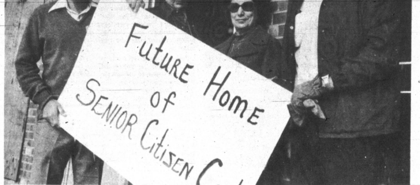
Starting Construction Work
