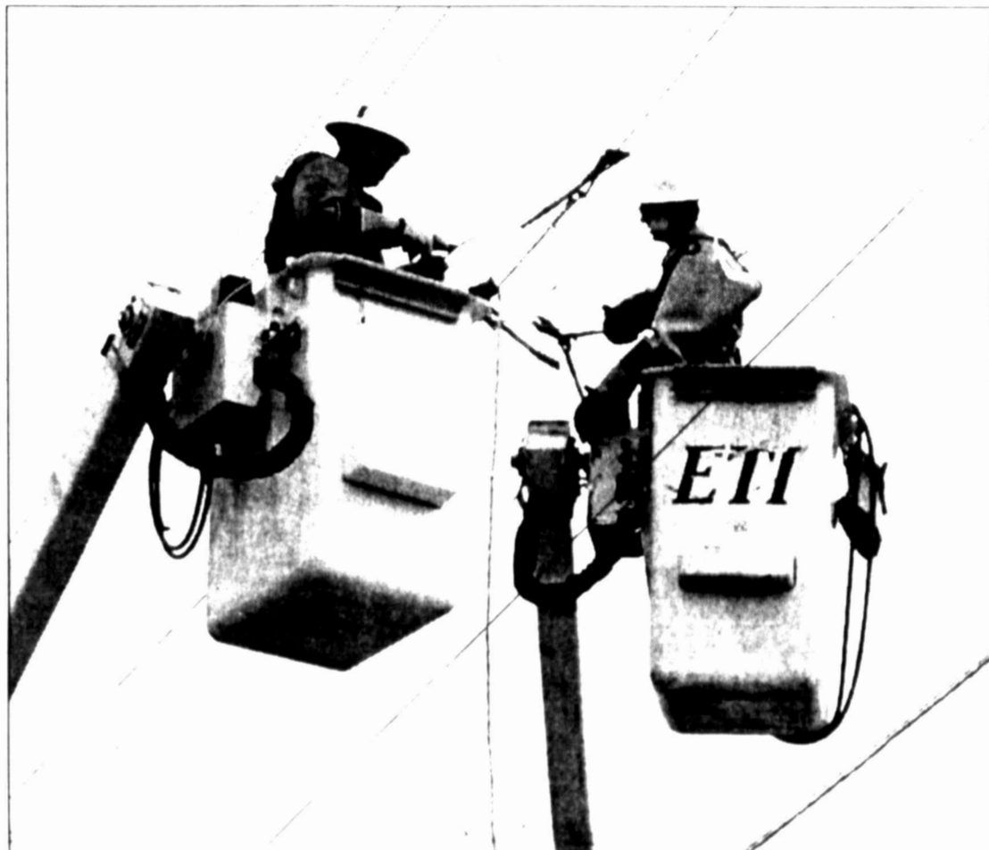
Oncor technicians Devry Kidd, left, and Nick Roberson work to repair a power line over FM 700 Thursday evening. The line was downed when a track excavator came into contact with it, causing a short circuit. The incident affected 697 customers, and left six, including Wal-Mart, powerless for about an hour.
