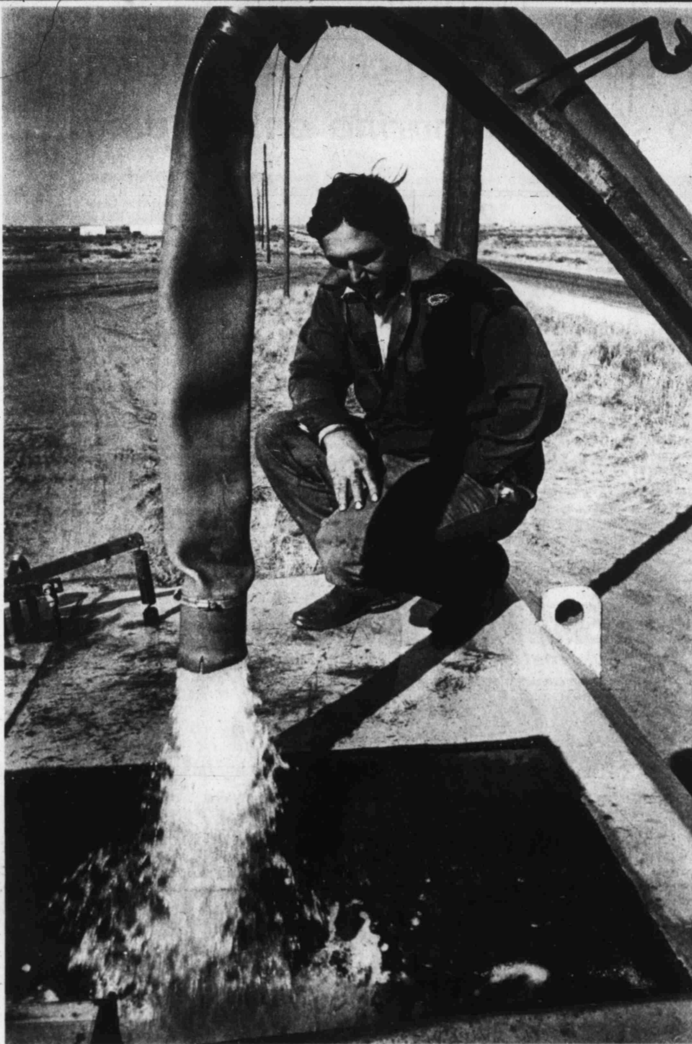
Running 3,560 gallons of water Monday for his water truck is Roy Horsey, who spreads water to cut down on dust and help pack soil ahead of earth scrapers and bulldozers at the Midland Park Mall construction site. The 750,000-square-foot
