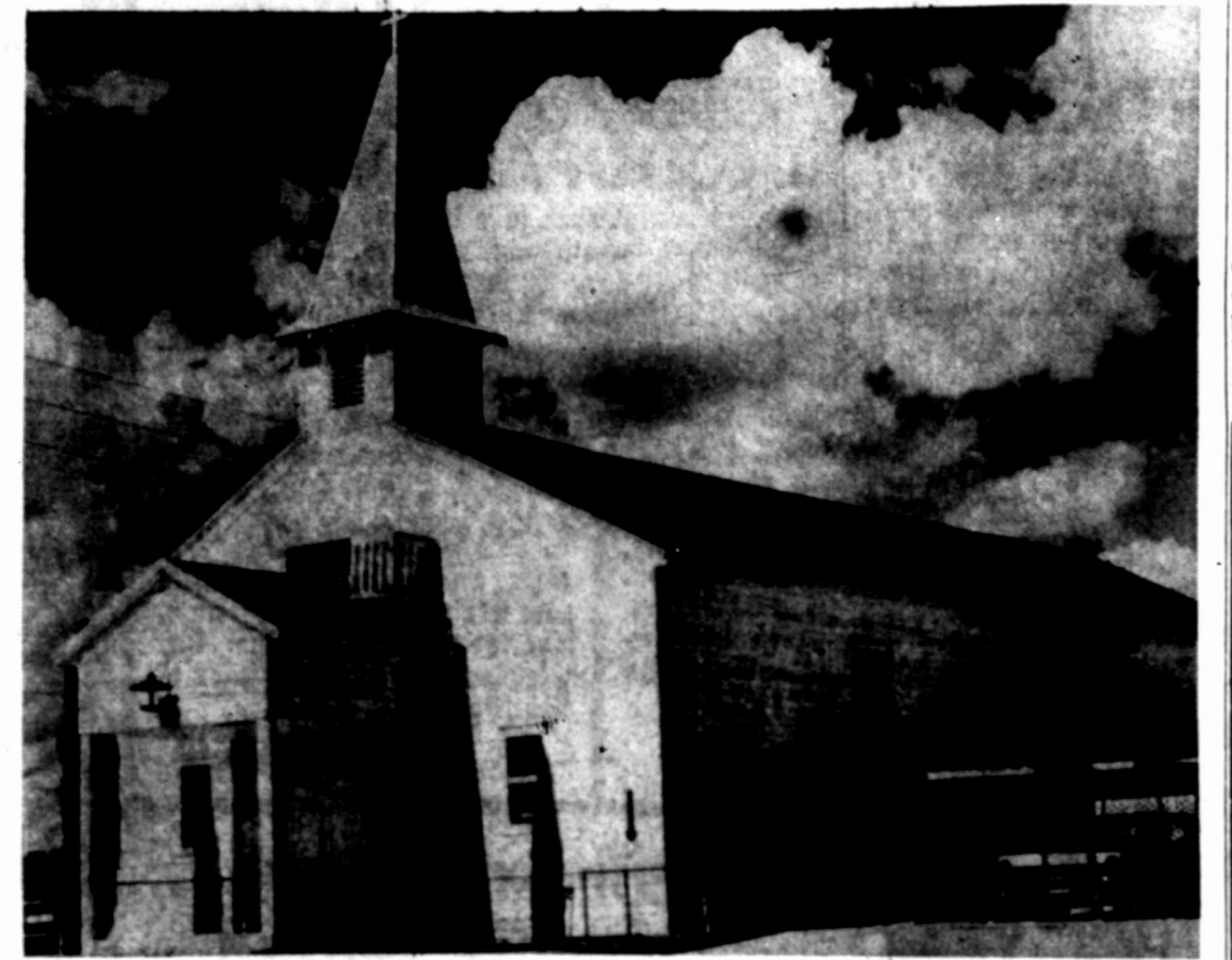
TO BE REPLACED when a new building is constructed is the Sacred Heart Catholic Church. The building was obtained from the base in 1946 and has been used by the congregation ever since. The Rev. Father James Delaney said construction will get under way on a new plant in October.
