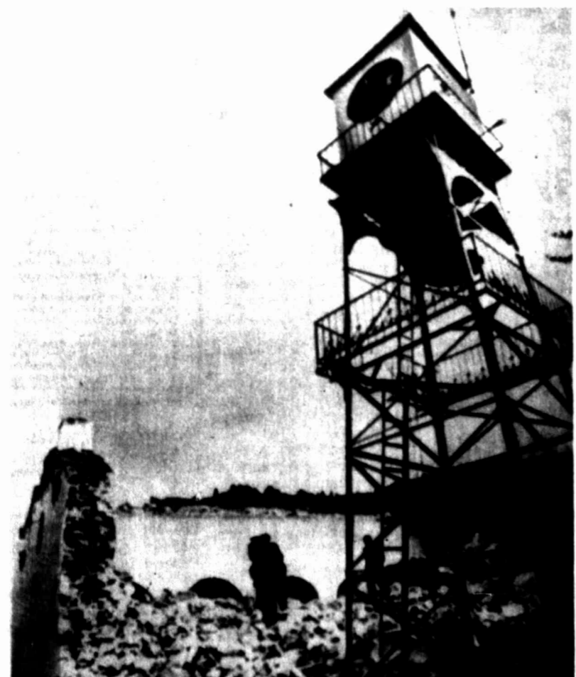
ALL THAT REMAINS — Only the bell tower remains standing in the rubble of a church hit by an earthquake at Perahora in southern Greece. A quake measuring 6.6 on the Richter scale struck the area Tuesday night, followed by another shock Wednesday morning.
