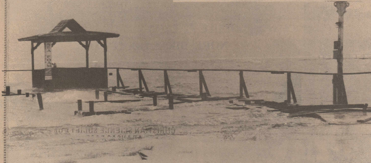
FLOODED-OUT PIER ON FULTON BEACH ROAD
