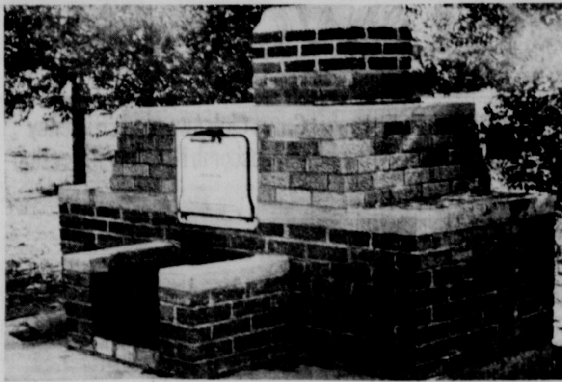
UNIQUE OUTDOOR FIREPLACE —One of the attractions of Friday's Ochiltree county home demonstration achievement tour was the above outdoor fireplace at the home of Mr. and Mrs. B. R. Pletcher, 618 S. Birch. Outstanding feature of the fireplace is the built-in oven which can be used for all types of baking.
