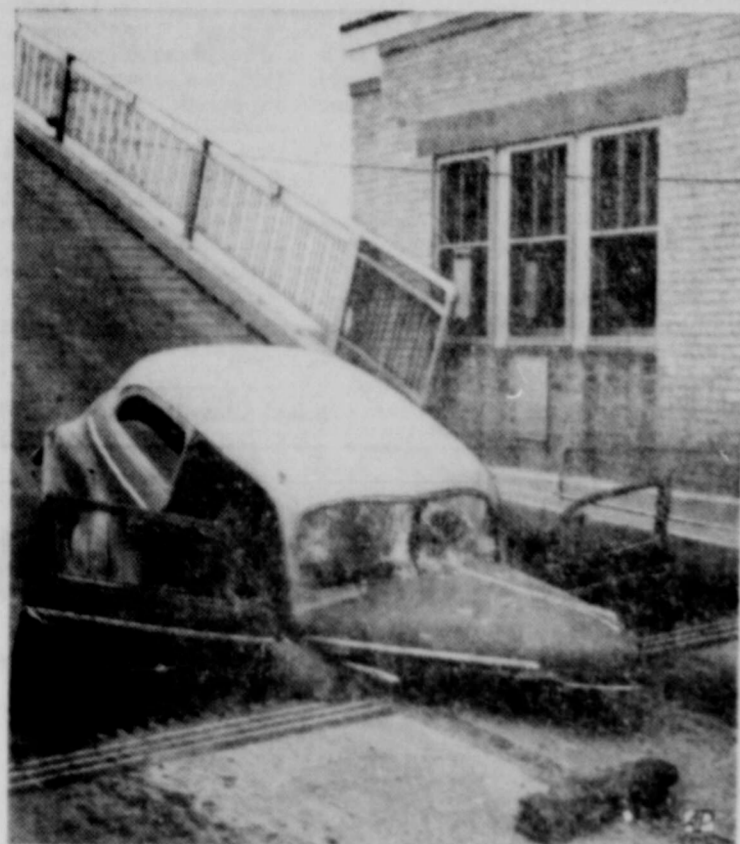
TOO LATE —This was the end of the trail for an automobile which claimed one rising span of Bascule Bridge over canal Port Arthur, surmounted its 50-foot length, jumped the gap where sections of the bridge split in the air, then raced down the opposite side, crashing into the concrete abutment. One man was killed in the accident and four others injured seriously. Operator in control house [right] cut off power to halt elevation of bridge as car began its wild climb after breaking through a barrier. (P) Photo
