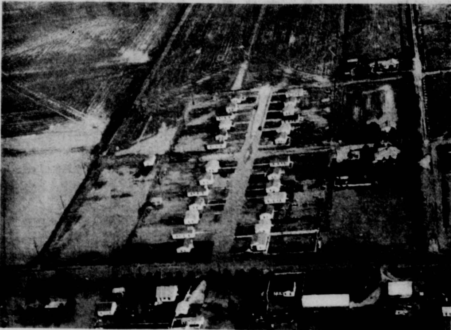
BELMONT ADDITION is virtually submerged in the above aerial photograph taken Tuesday morning after some water had already drained from the area. (Herald Staff Photo Engraving) (Flight Courtesy Omar Truax)
