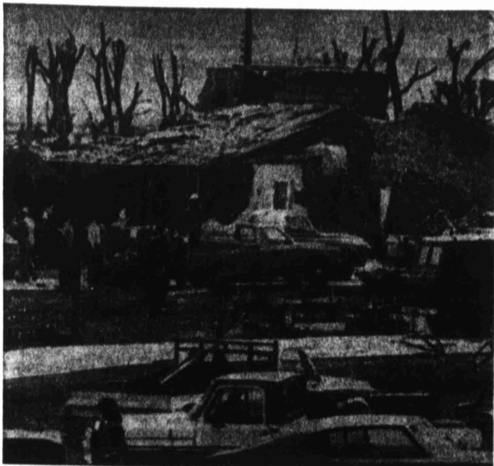
TORNADO CLEANUP —Residents and friends came from all around to help those whose homes were destroyed in a killer tornado which struck Plainview Sunday morning. The Forest Mickey home (shown) was located in the fashionable Westridge section of Plainview.
