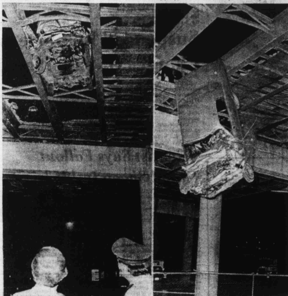
SAVED BY INCHES — Houston police officers, left, look at a car that drove off Interstate 45 in the downtown area, sailed 32 feet through the air and came to rest between two steel girders in a section under construction. Two hours later, after the occupants had been removed, the auto falls onto a parking lot. The driver was charged with DWI. (AP Laserphoto)
