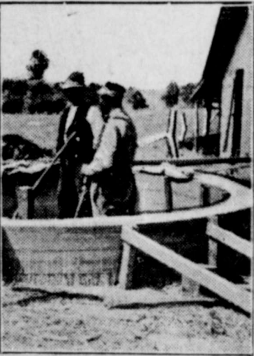
Laying the Foundation of a New Silo.
