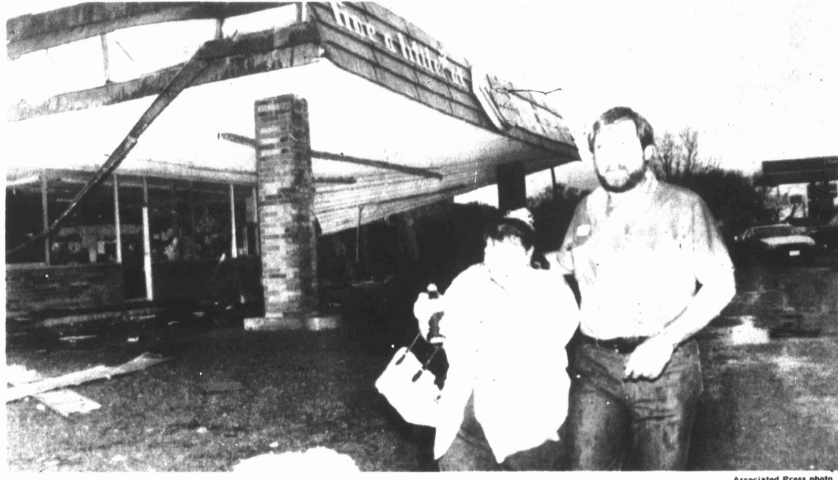
CHANDLER — Melinda Little, left, and Jim Palady leave the scene of destruction caused by a tornado which swept through Chandler, a small town west of Tyler, Tuesday morning. The twister damaged a Dairy Queen and several office buildings, causing two injuries.
