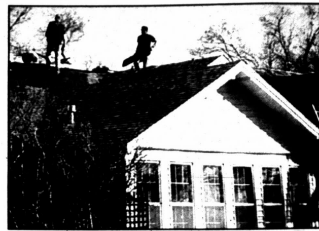
Employees of Wendell's Roofing Co. as they enjoy the spring-like weather while replacing the roof at 1020 Mary Ellen.
