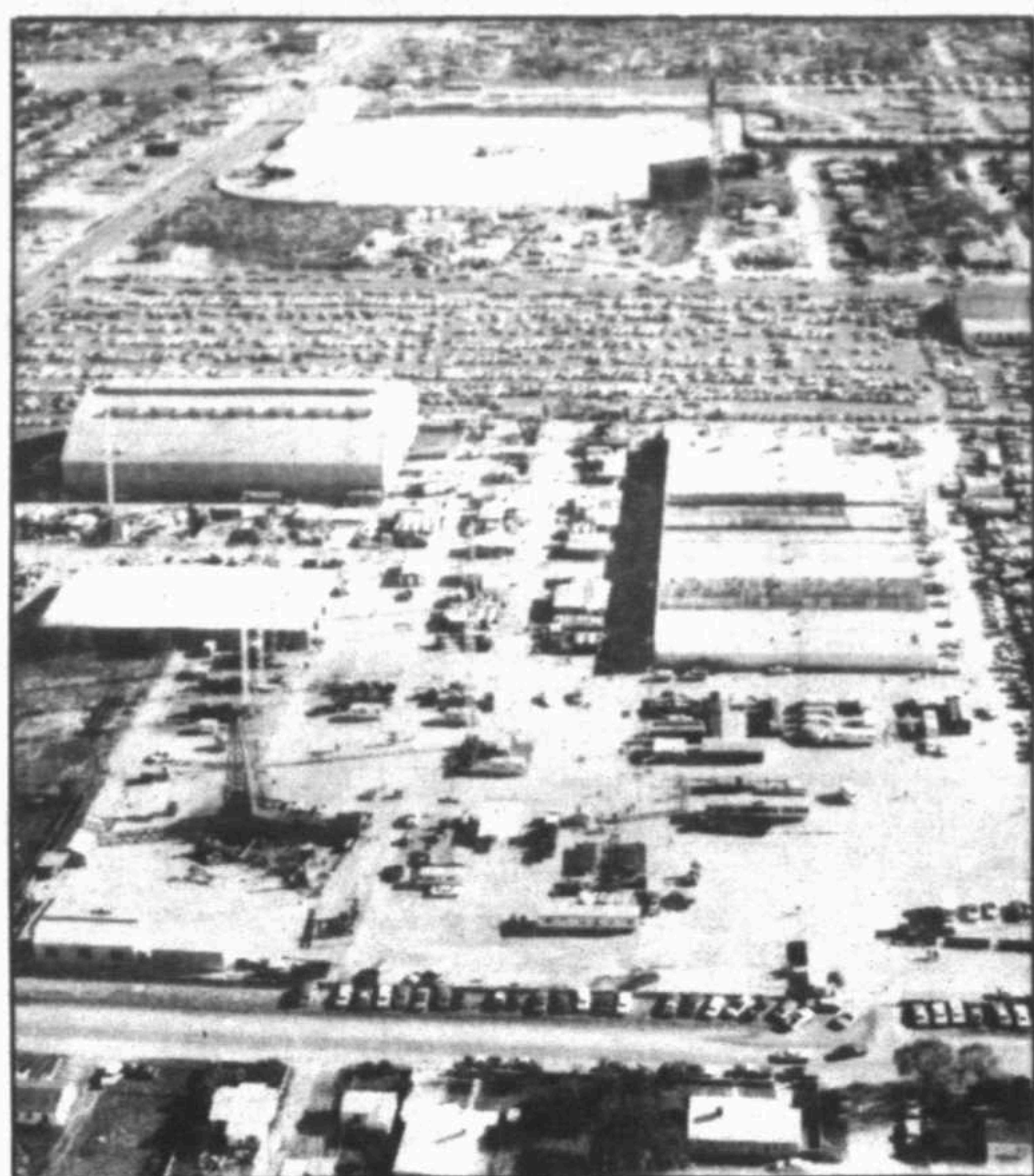
Both the Oil Show and the neighborhood have changed in the past 30 years. This year the show will take on an even better look with newly renovated facilities.
