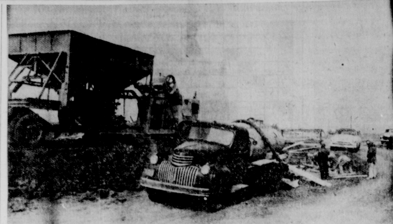
BOOKER FARM ROAD—Bell and Braden construction crews are pictured above completing a bridge on a new farm to market road which runs from the Oklahoma state line north of Booker to a point several miles south. All dirt work on the road has been completed and structures should be finished in the next ten days according to W. O. "Bob" Mauldin, foreman on the project. The road will likely be topped next spring Mauldin said.
