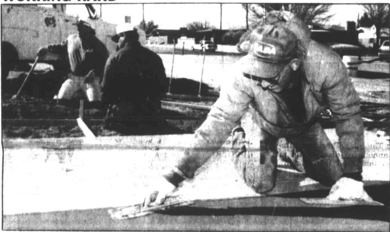
With others working in the background, school district employee James Norman smooths out concrete in front of Goliad Middle School Thursday. The work is being done to bring the schools into compliance with the Americans with Disabilities Act.
