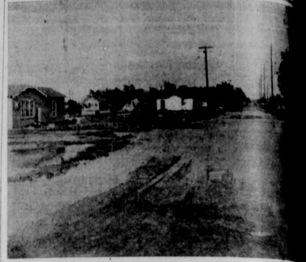
NORTH SIDE FLOODED —This street scene, taken in the residential district in north Perryton shows how heavy rains have completely inundated the area.
