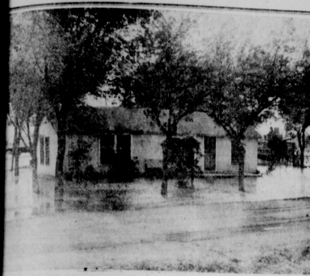
ER BOOTS—This is the R. M. Morris home, across the street west of the power plant, which is completely surrounded by water since the Sunday night rain.
