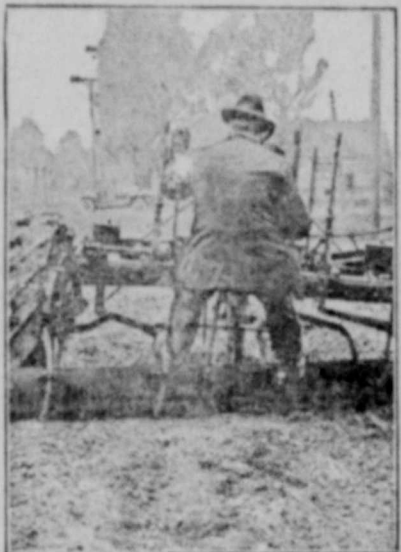
A Modern Implement for Smoothing Dirt Roads.
