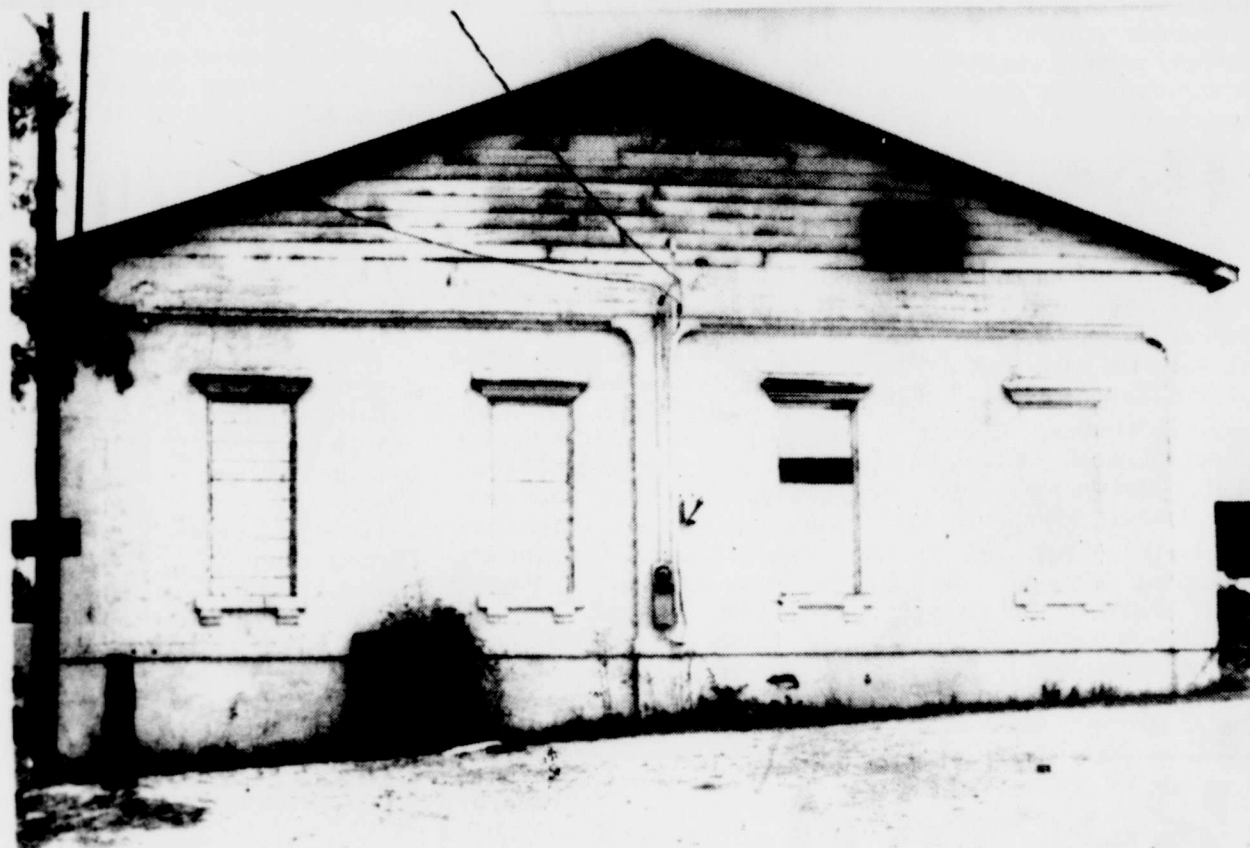
THE VETERANS OF FOREIGN WARS building was gutted by fire Wednesday night. Interior fire damage was confined to a bathroom and hallway on the east side of the building, with smoke damage found throughout the structure. There were no signs of serious fire damage on the exterior. Fire Marshal Billy Ray Williamson said an investigation to determine the cause is still under way. VFW officials could not be reached for comment Friday.
