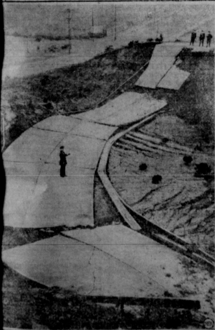
Public evidence of the tremendous force of the landslide which tumbled down from Lone Mountain, San Francisco, is offered by this wreckage of concrete roadway, twisted apart and flung in huge blocks 60 feet from its original position. Sidewalks and pavements buckled, telephone poles snapped, and the San Francisco College Women veriled, the enormous slide starting only 60 feet from its buildings.
