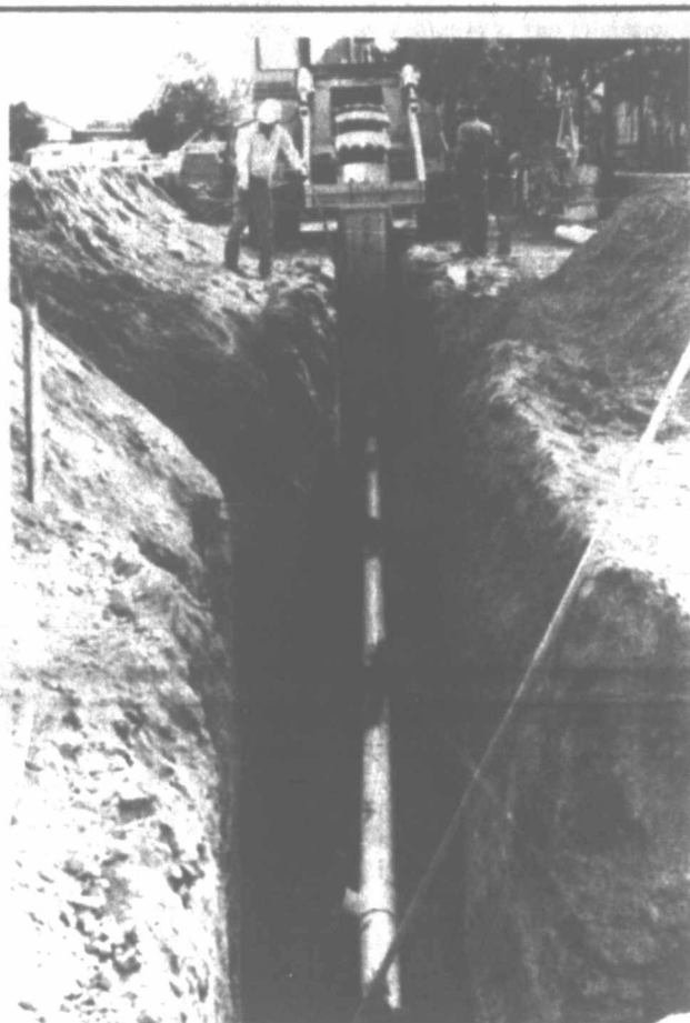
The project includes installing 13,700 feet of pipe. The contractors say the job has been slowed somewhat by recent rains and by having to dig through rock in places. Sub-contractor is HBH Construction of Odessa.
