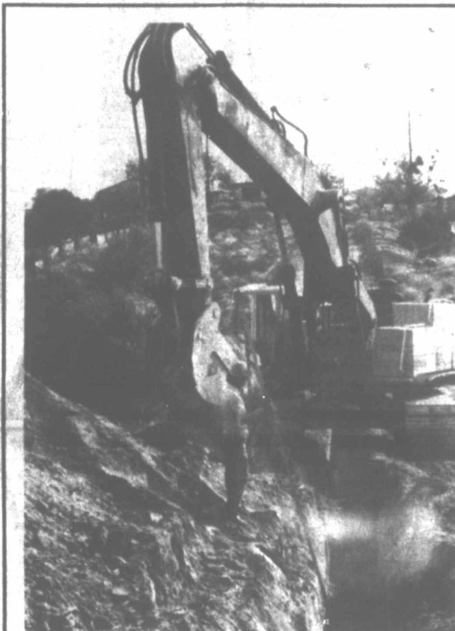
CONSTRUCTION is continuing on the installation of sewer line in the north part of town. Contractor for the job, funded with a grant from the Texas Community Development Program, is Panhandle Construction.
