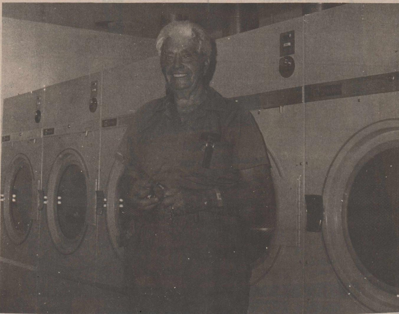
DON ADAMS OF DON ADAMS LAUNDRY is shown here with a few of the 7 new dryers just installed at the laundry.
