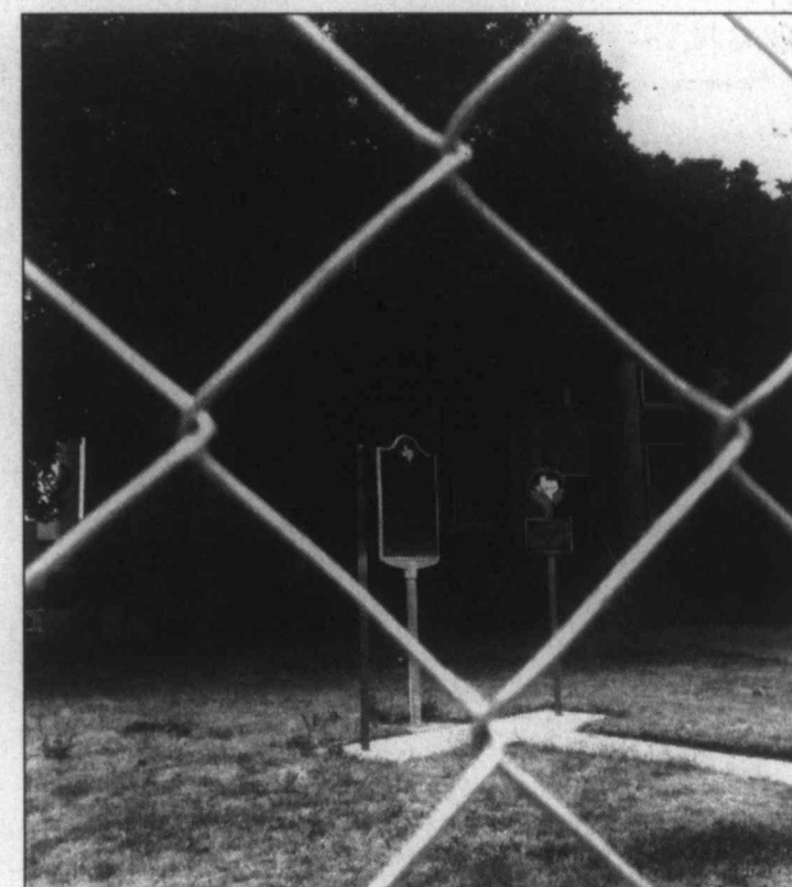
No public allowed... Chain link fencing has been placed around the Lynn County Courthouse, as renovation work is underway on restoring the historic building back to its original look from 1916, both inside and out. A Texas Historical Commission grant through the Courthouse Preservation Program is helping fund the $8.5 million project. The courthouse will remain closed for the duration, most likely 18-24 months. All county offices have relocated to new temporary office locations in Tahoka. (LCN PHOTO by Juanell Jones)
