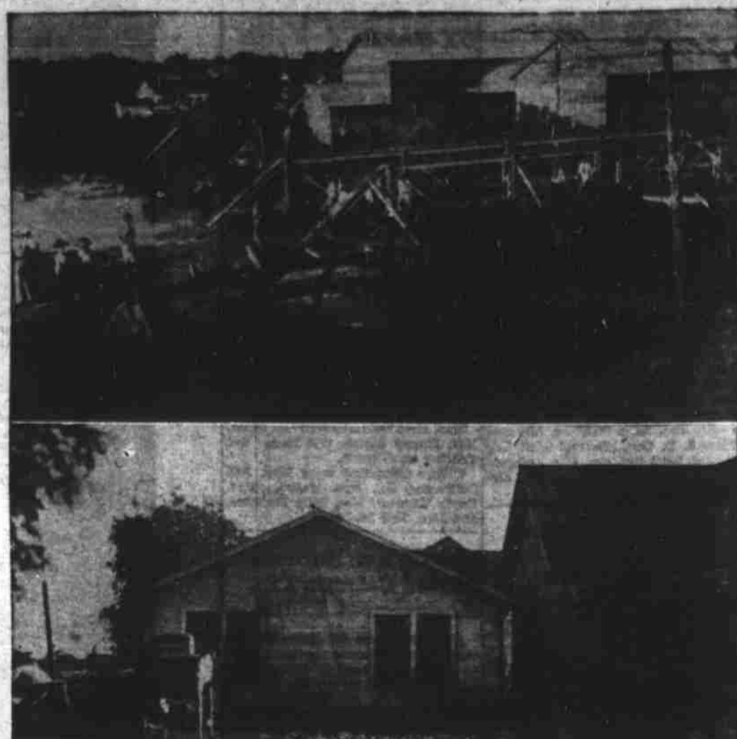
Sights Snyder people never expected to see were left by the flooding Deep creek, in the west edge of town. Two of them are shown above. In the top picture debris is seen stacked high on a bridge on the highway leading toward Gall. (Two blocks farther downstream a similar bridge was washed out.) Left in the lower picture is the home of T. J. DeShazo, night watchman. While DeShazo night watched, and his wife, daughter, son and son's wife barely made their escape, Deep creek spun the house all the way across the street and parked it against the residence of Ivan Teeter as shown. (Ahlene Reporter-News photos).
