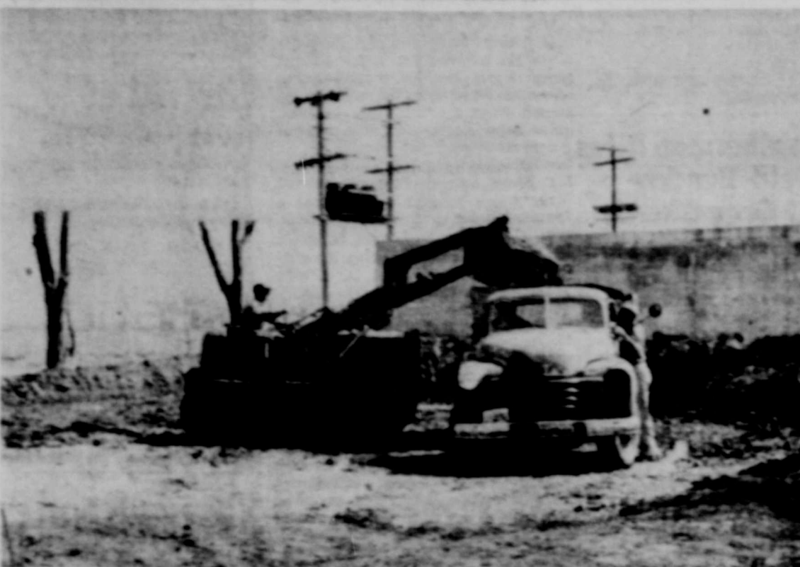
NEW RESERVOIR—Work has begun on constructing the new 250,000 gallon concrete water reservoir for the city and this truck is being loaded by equipment of the Ferguson Ready-Mix Co., who received the construction contract. The reservoir, of reinforced concrete, will be built for $10,400, amount of the Ferguson bid.
