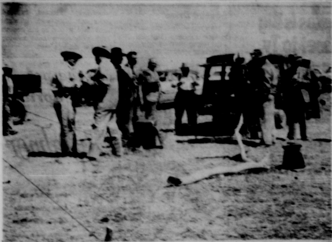
NOONTIME—Members of the bridge dedication committee from Roberts, Gray and Ochiltree counties met Tuesday at the bridge site on highway 70 to make plans for the April 29 dedication. They were served barbecue by Frank Carter of Pampa and about 50 men took part.
