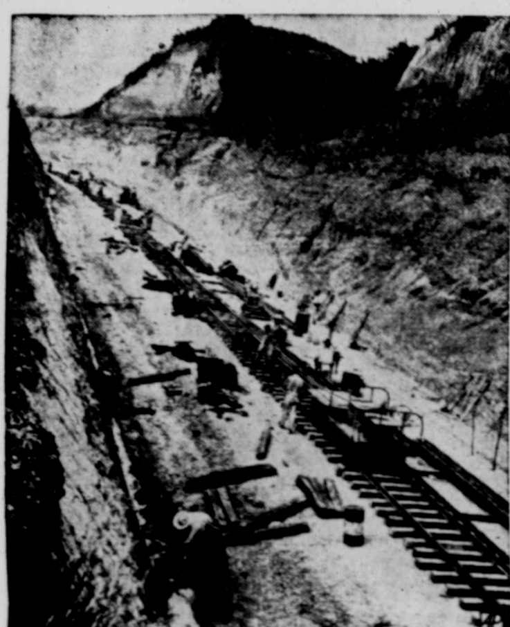
DOWN IN THE VALLEY — Workmen lay rails during construction of section of 600-mile rail system in Colombia's Magdalena River Valley. Target date for completion is 1960.
