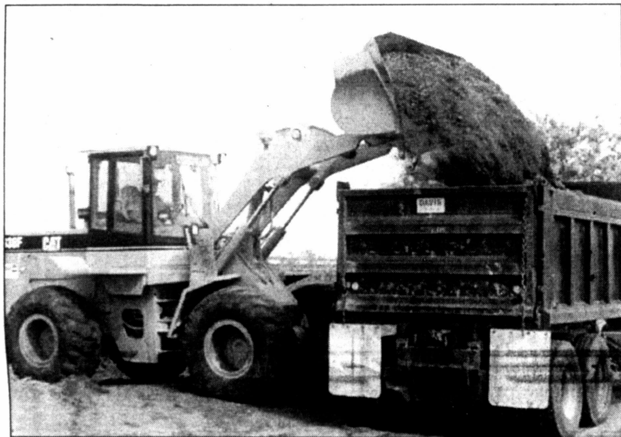
PCT. 3 CREWMAN John Morris was loading dirt into one of the county dumptrucks that was hauling dirt from west of the Wallace-Ware Units to the construction site of the new hospital and physicians' clinic. Supervisors expected to need 300 truckloads to move more than 13,000 cubic yards onto the site.
