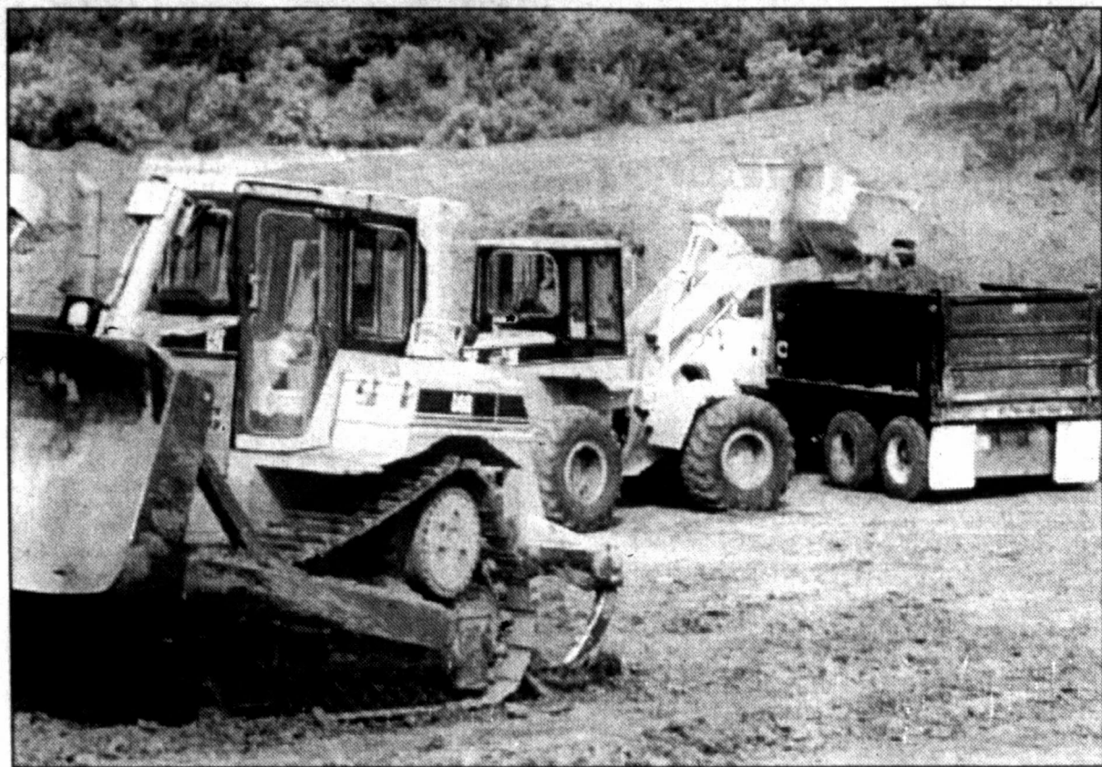
COUNTY ROAD AND BRIDGE CREWS were loading soil with a high clay content on the east side of the Colorado River near Interstate 20 last Thursday, having resumed work Wednesday to prepare the nearby Mitchell County Hospital site for construction. The dug out area on TDCJ property west of the prisons here will be used to create a tank, or pond.
