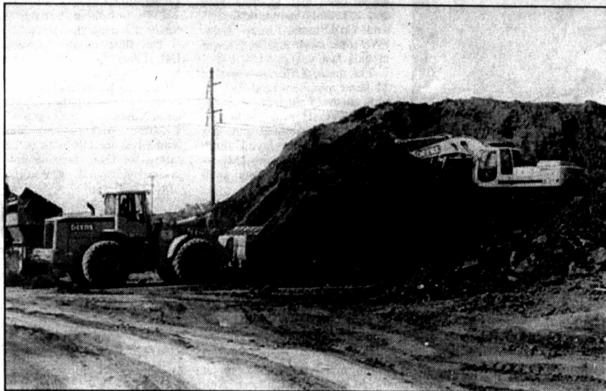
FEEDING THE SCREENER with hydrocarbon loaded soil is a fastpaced job for the Lone Wolf Resources loader driver on the left, who also scoops gravel from another pile where LWR is cleaning up the old Coltex Refinery site southwest of town.
