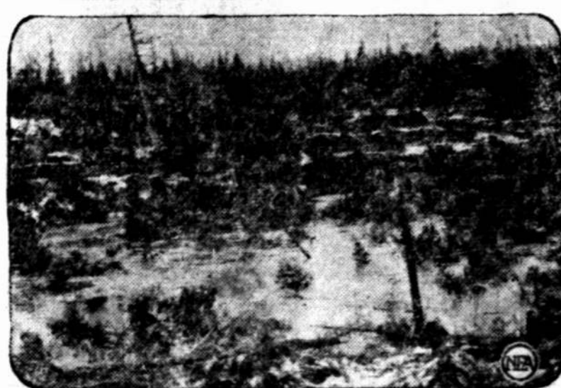
Six acres of ground sank into this morass when an underground lake burst through walls of the Baross-Hoeker iron mine at Ishpeming, Mich., a quarter of a mile distant, and drowned 51 men. Banks around the edge show how the earth collapsed.
