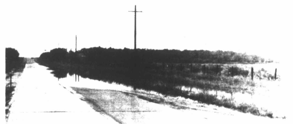
Water From Emergency Spillway At Lake Colorado City Flows Onto Hwy. 163
