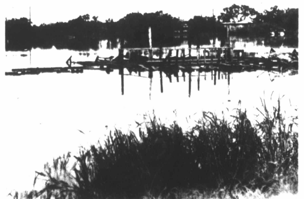
One Of Many Boat Docks Destroyed By Flood Waters At Lake Colorado City
