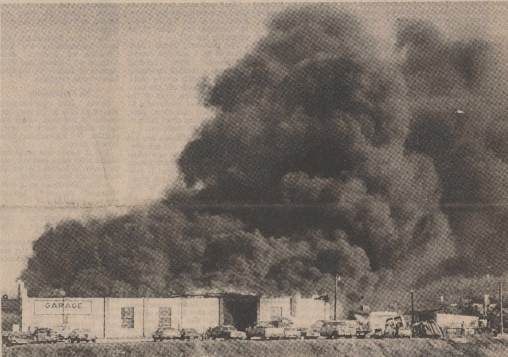
Flames cover roof
