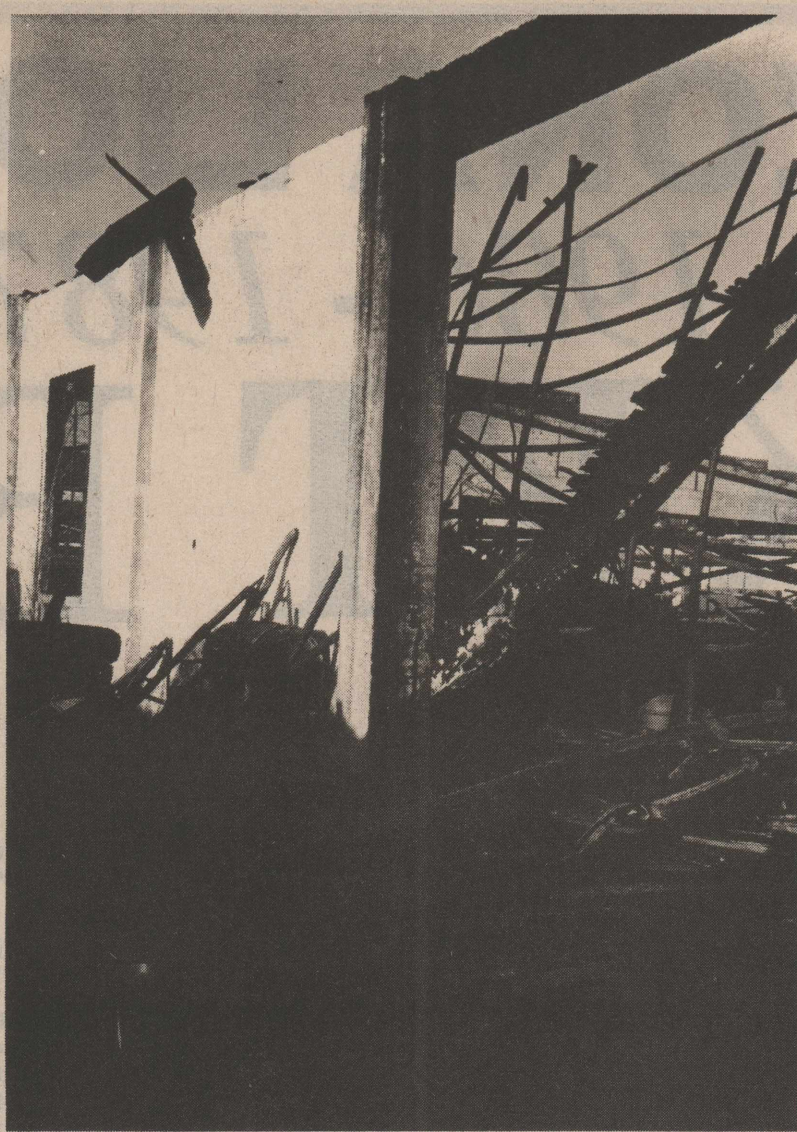
THE AFTERMATH of the fire which destroyed Skains Motor Co. There was nothing left but rubble and a clear blue sky Sunday afternoon, but smoke was still rising from the ashes.
