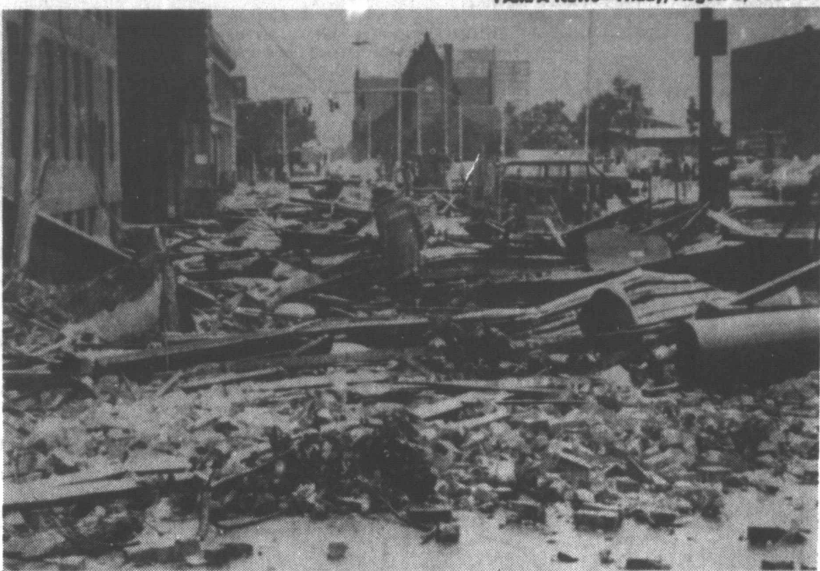
TORNADO DAMAGE — A lone firefighter walks through rubble outside a factory building in downtown Providence, R.I., Thursday afternoon in the aftermath of a
