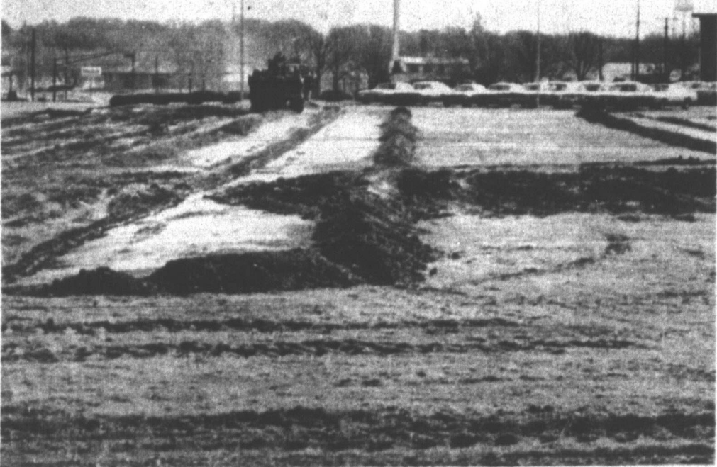
ON THE LAST STRETCH—Workmen have begun to grade the area for the parking lots for the M.K. Brown memorial auditorium as construction enters the final phases for the April 23 dedication date. Workers of the E.D. Baker Construction Co. of Borger are grading an area north of the auditorium to prepare it for later surfacing. Plans for adjacent street paving have also begun.
