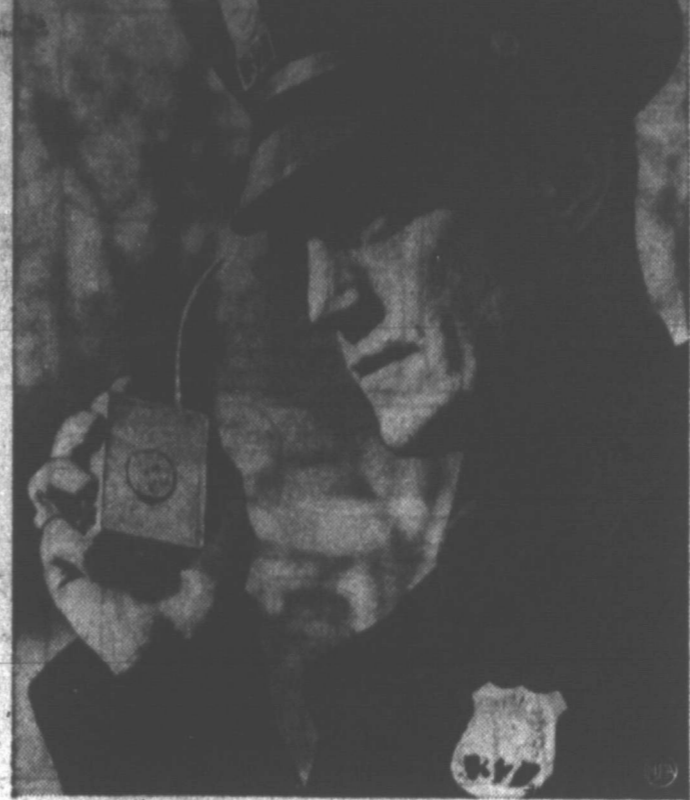
LISTENING POST—Patrolman Raymond Beardsworth of the Bridgeport, Conn., police department receives instructions from headquarters via this newly developed radio receiver. It is called the "cigaret pack" radio and was developed by Clifford F. Fraser, police communications supervisor. The receiver is operated by subminiature tubes from low battery current and reception is good up to 40 miles away from the transmitter. It is not designed for two-way transmission.
