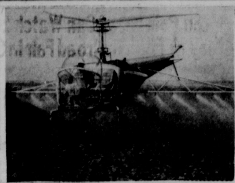
WEED-KILLER—This helicopter flying, 40 miles an hour, 10 feet above the ground, sprayed a 170-acre wheat field near Dodge City, Kansas in an agricultural demonstration.
