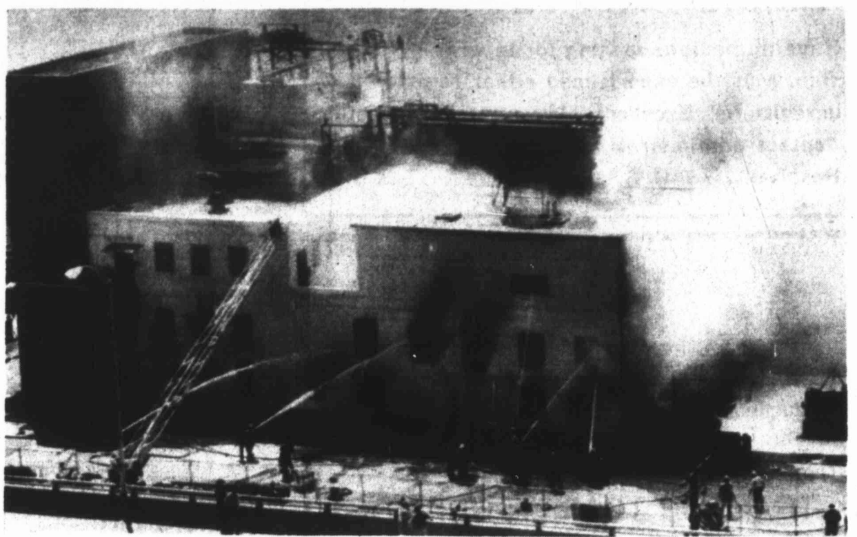
REFINERY FIRE — Firemen battle a fire in the wax section of the Ashland refinery in Freedom, Pa.
