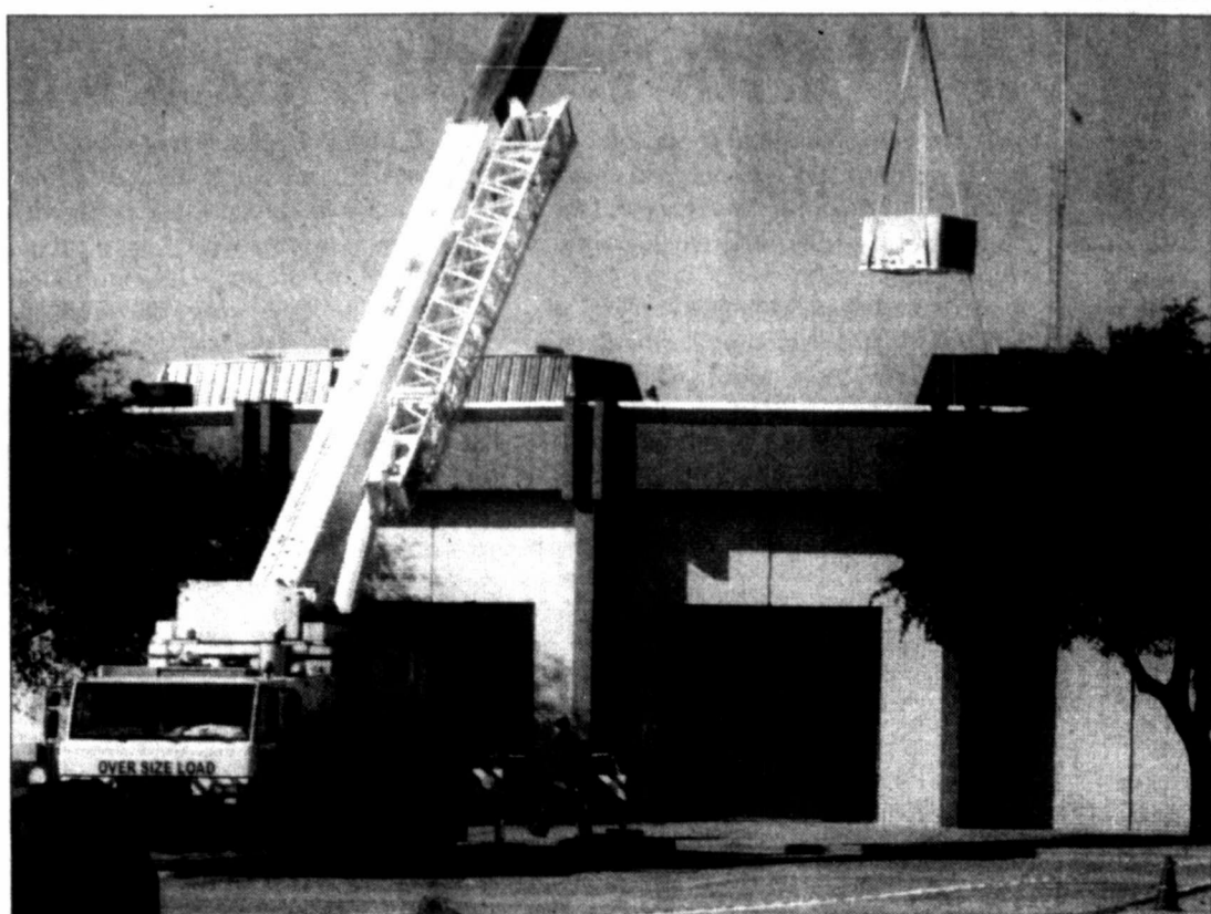
NEW AIR CONDITIONING AND heating units are going in all buildings at Colorado High School starting last week. The outer buildings are being installed in the coming weeks, with the main building being installed while students and teachers are out for spring break.
