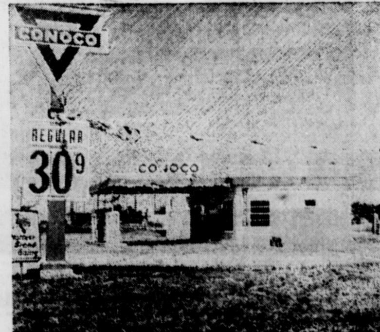
THOMPSON'S CONOCO STATION — Located on East Highway 80 will hold their reopening on Saturday, April 27. (Staff Photo)
