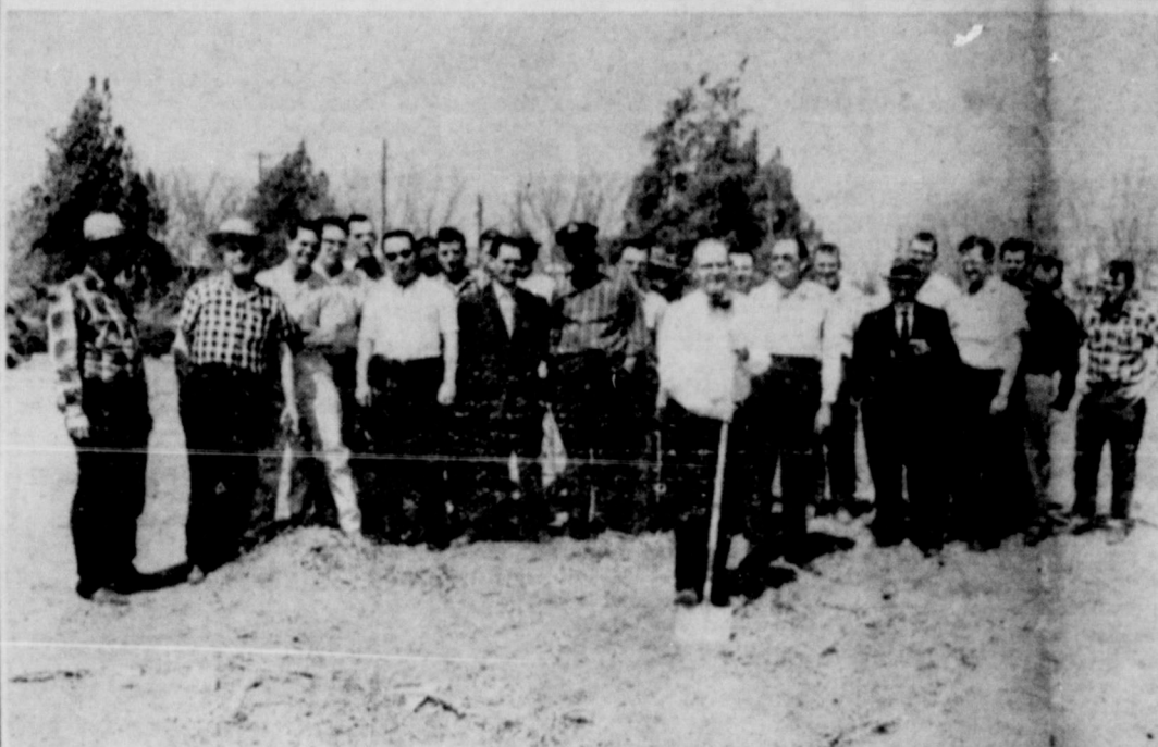
GROUND BREAKING — Lion John G. Robbins is shown turning the first spade of dirt at the swimming pool site. In the background are members of the Lions Club.
