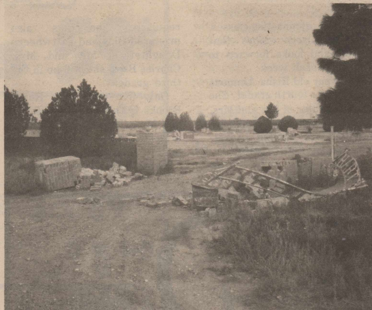
GATEWAY DAMAGED - The ironwork sign and brick columns which support it at Hart Cemetery were knocked down last weekend. Investigation is underway by Castro County Sheriff's Department.
