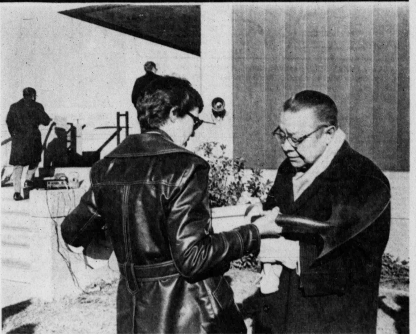
Frank Stubbeman, immediate past president of the Midland Memorial Foundation board of governors, signs a shovel used in-groundbreaking ceremonies this morning for renovation and expansion of Midland Memorial Hospital public
