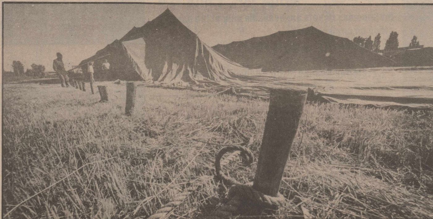
4. Side Poles Are Set At End, And . . . .
