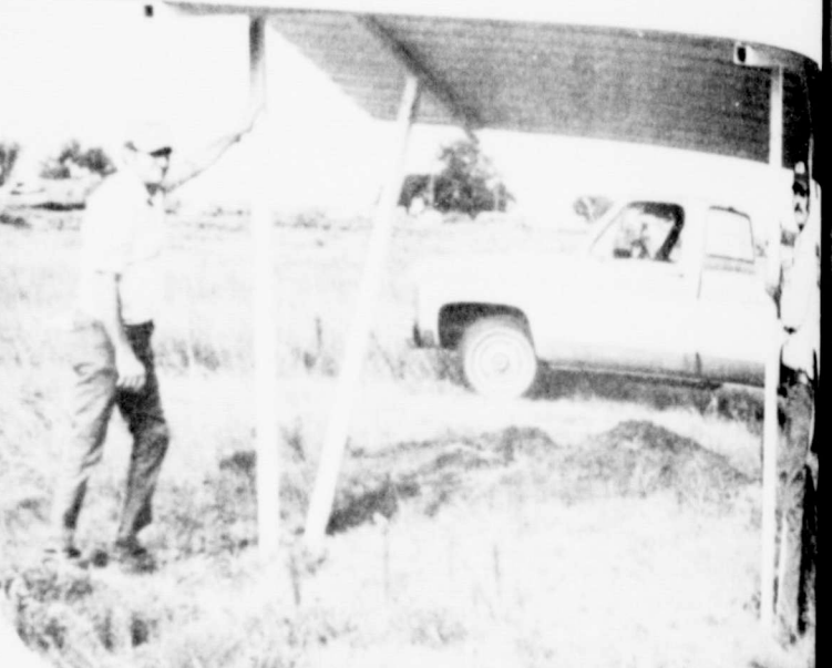
KIWANISANS Corky Guffee and Jerry Neeley install a sign at two parks last week. Russell's Equipment made the sign.
