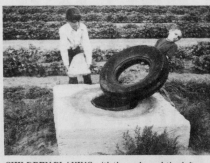
CHILDREN PLAYING with the rocks and tire left as a "cover" atop the cement block of this abandoned well. The District urges farmers to cap abandoned wells in such a manner that children at play cannot lift the cover and expose the open hole.
