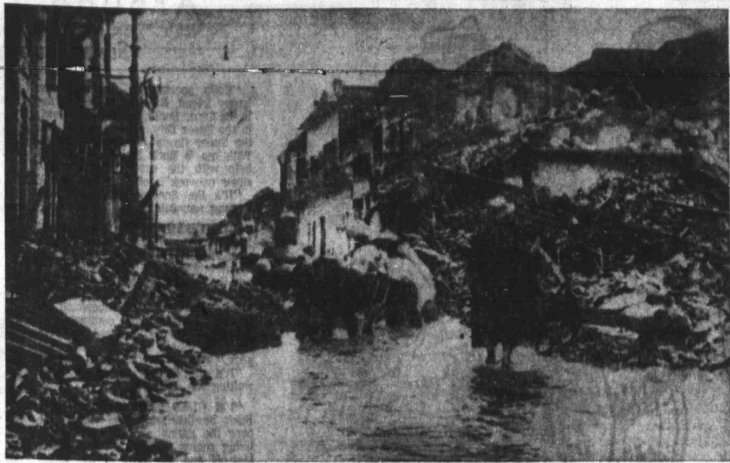
Workers Clear Debris-Clogged Street
