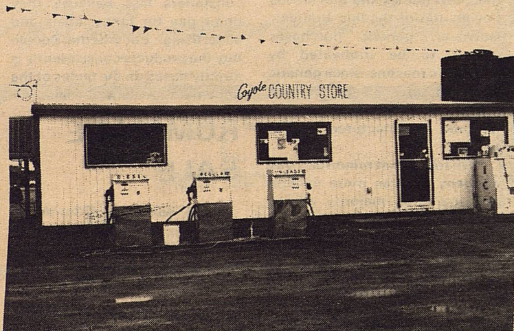
THE NAME OF THE NEW STORE AND STATION IS VERY APPROPRIATE-THE COYOTE COUNTRY STORE.
