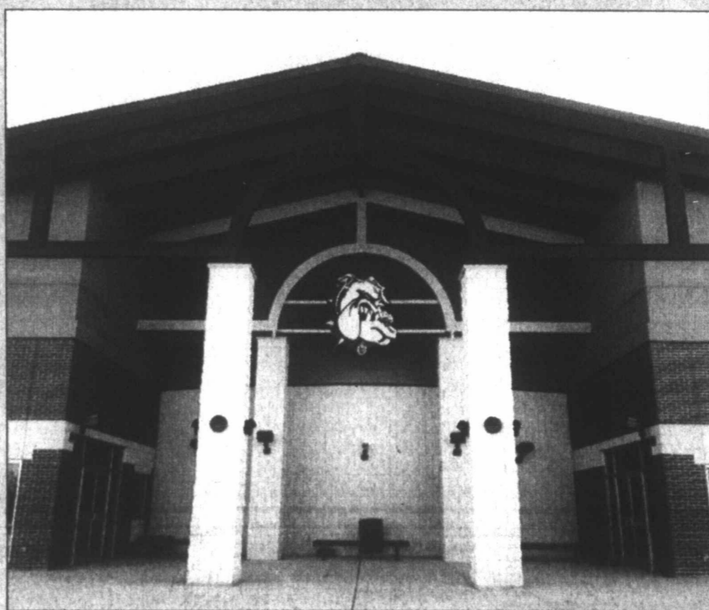
BULLDOG PRIDE - Work on the newly constructed Loraine ISD campus is complete and school officials are brimming with pride. An open house and dedication ceremony will be held on Saturday, August 24th. Photo courtesy of Travis Edwards.
