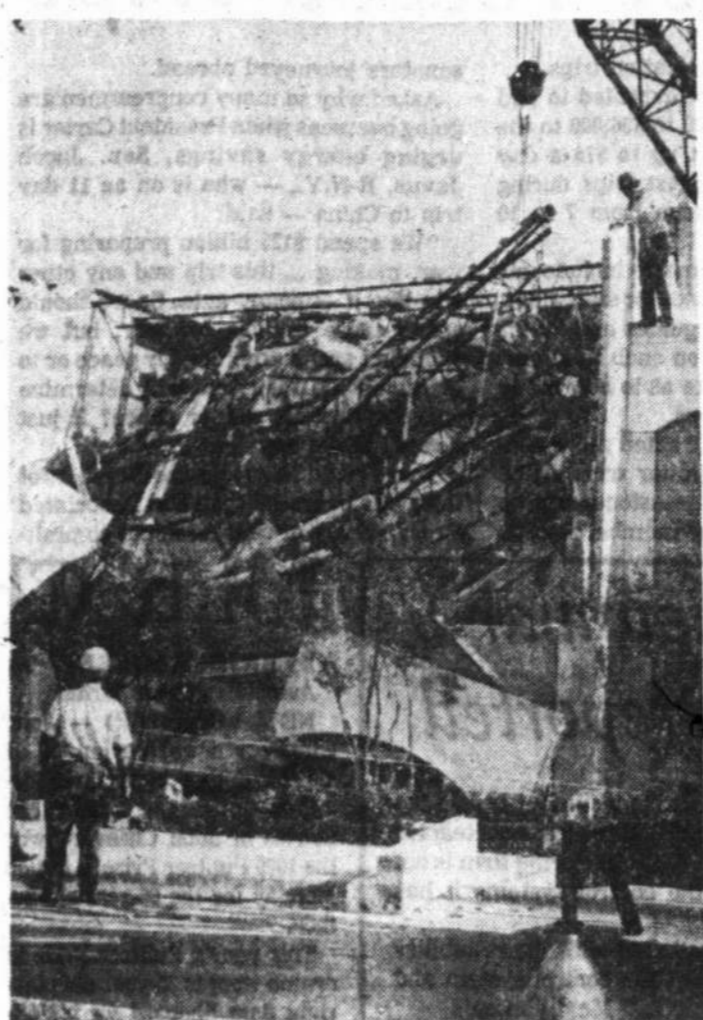
Portion of wall at Wichita Falls Museum and Art Center collapses during repair attempts (Photo by J.G. McCall)
