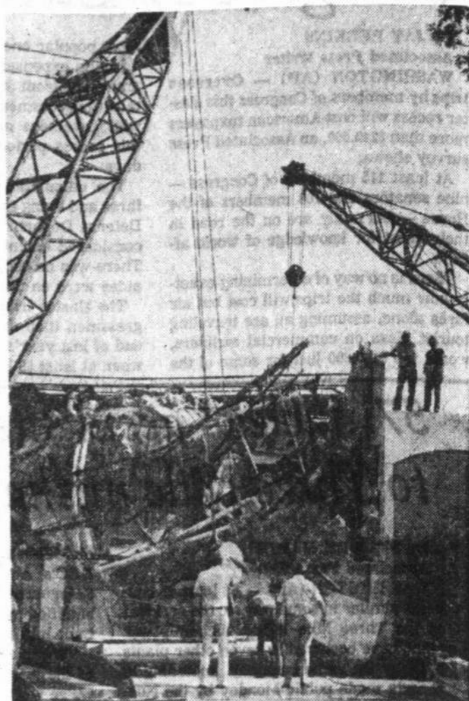
Portion of wall at Wichita Falls Museum and Art Center collapses during repair attempts (Photo by J.G. McCall)
