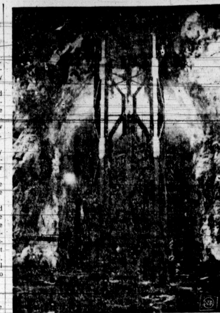
HOLDING UP A MOUNTAIN —Seventy-foot-tall steel beam jack holds up the ceiling in one of the subterranean chambers hollowed out inside Cheyenne Mountain near Colorado Springs, Colo., for the North American Air Defense Command's new combat operations center. The jack will hold rock in place until repairs can be made with steel and concrete. A three-story building will go in this section to house the NORAD command post where information from air and space detection networks across the continent will be displayed.
