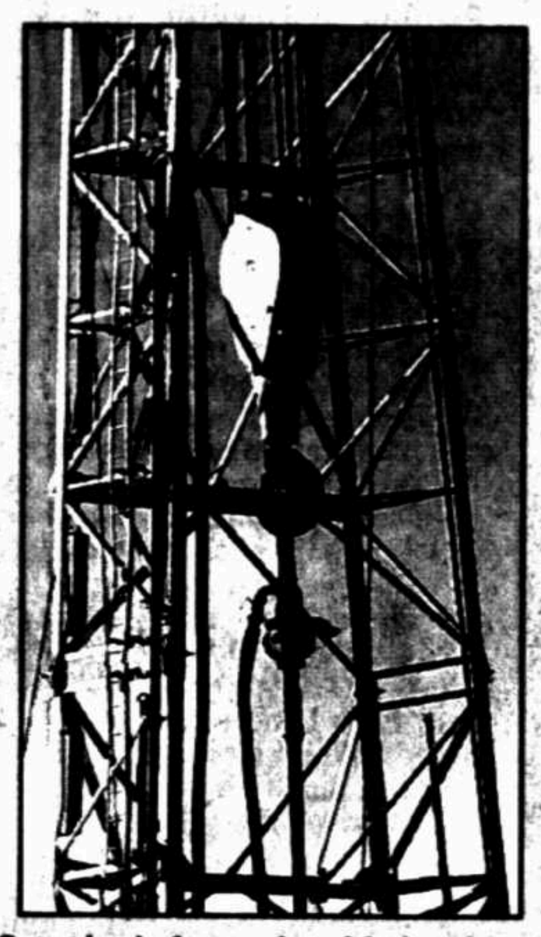
Seemingly frozen in mid-air, a block makes its trip up the derrick. This week's rig count dropped slightly to 137.
