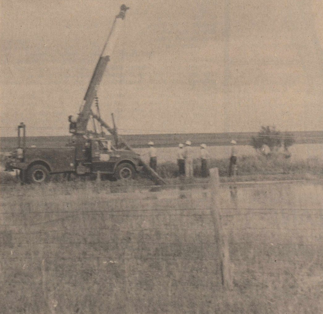
REPAIR WORK BEGINS--Electric company employees begin repair work on lines downed west of Circle Friday after Thursday night storms left heavy damage to crops in the vicinity. Up to six inches of rain was reported during the storm.
